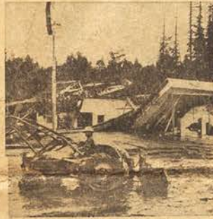
With a scene of utter destruction as a backdrop, this tractor operator undertakes the gargantuan task of clean-up in the battered town of Weott.
