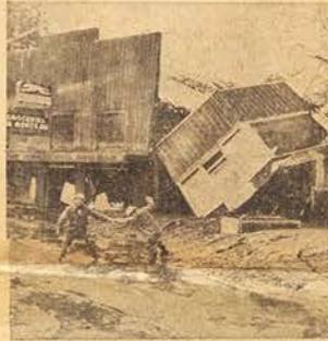
Swiftly flowing flood waters flipped the Weott post office over on its side during the disaster. Ankle-high water remained on the downtown street for several days afterward.
