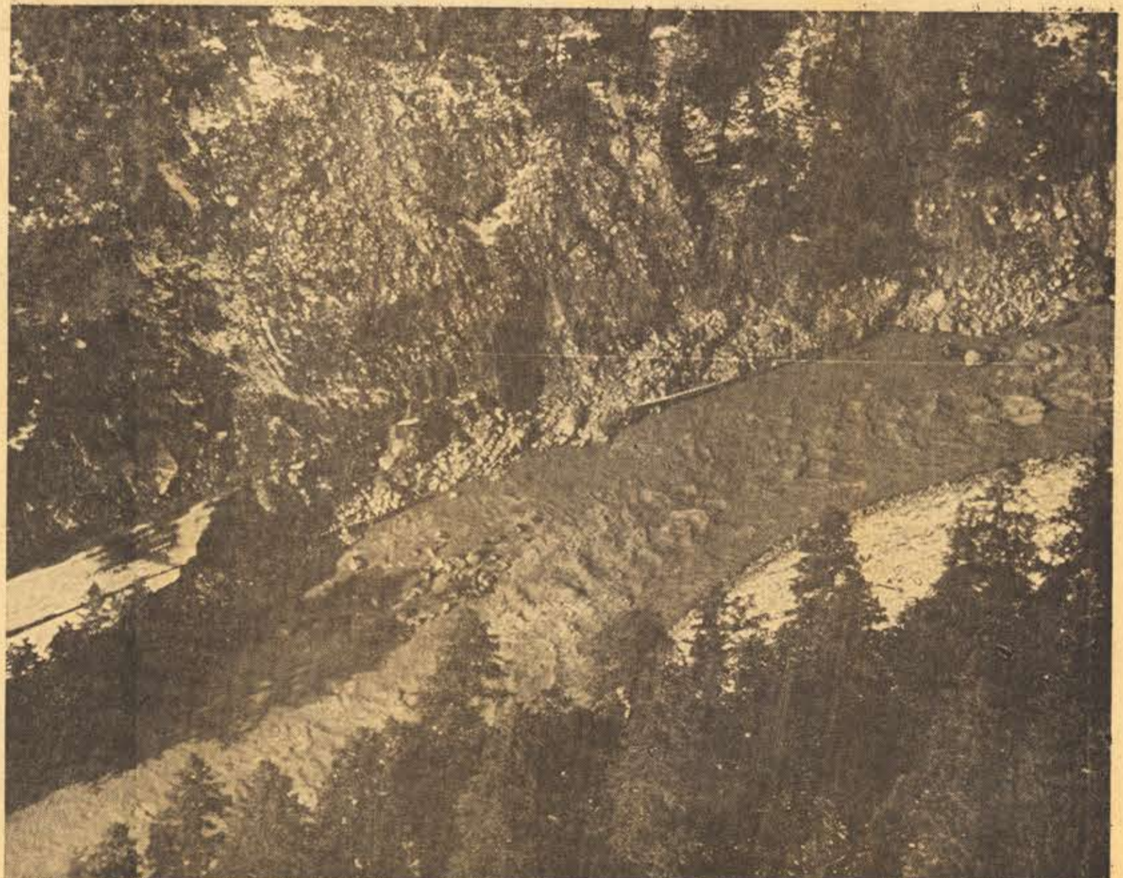
Christmas week flooding wiped out 12 and five-tenths miles of Highway 199 east of Gasquet in Del Norte County. Note the battered section which remains (left).
